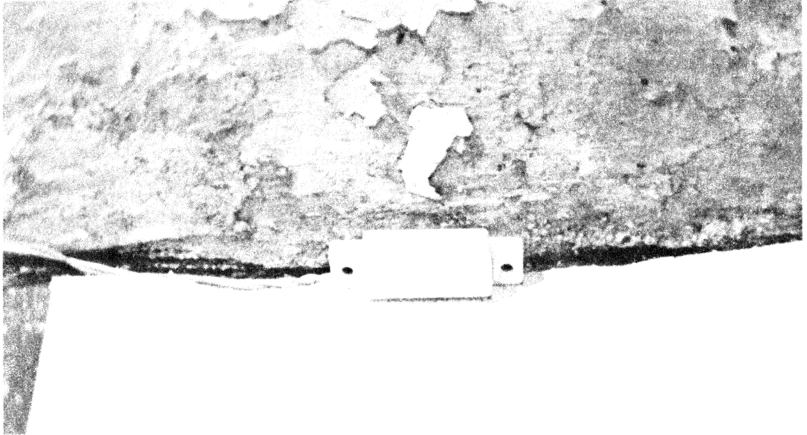
Fig. 18-23. If the basement floor becomes flooded, this moisture sensor will detect the condition. Note the paper towel used to absorb water and speed detection.
